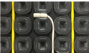
Mark the positions of the floor fitting objects that will be installed once the floor is finished, so these can be avoided when laying the heating cable.
